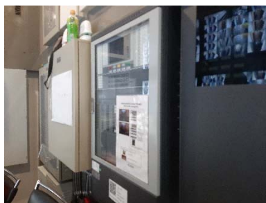
Graphic Annunciator Fire Alarm System
