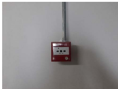
Fire Alarm Manual Station
