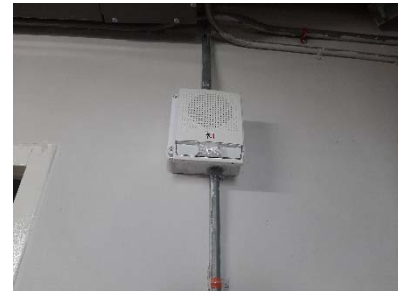
Fire Alarm Horn Strobe
